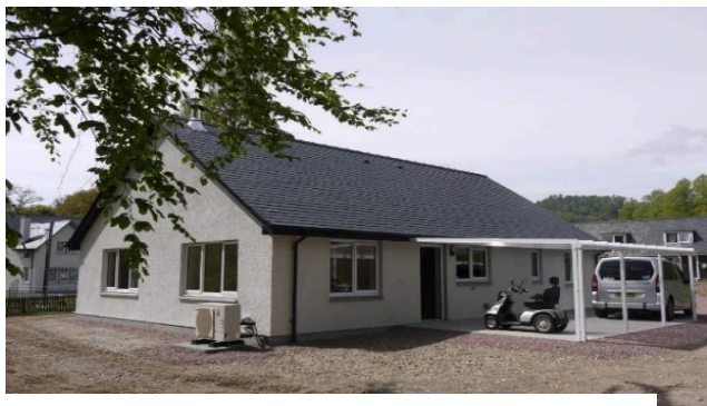
CHT Adapted Built home, Invergarry.
